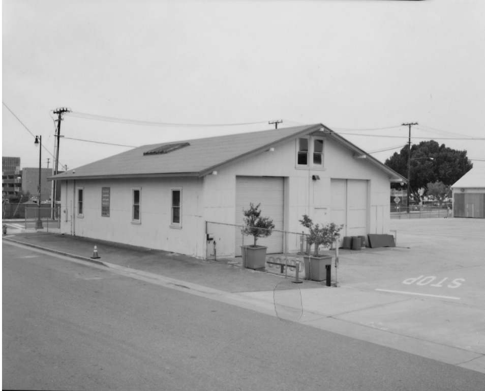
Figure 13 Building 3, facing southwest; Photograph by Tavo Olmos, 2014
